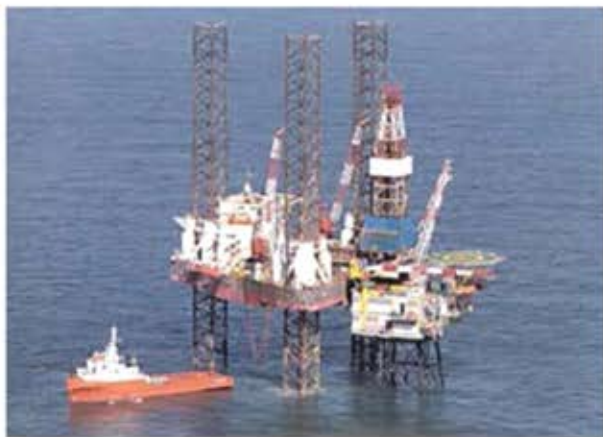
© Wintershall Q4-C platform, North Sea
