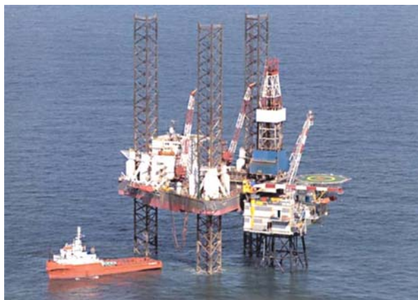
© Wintershall Q4-C platform, North Sea
